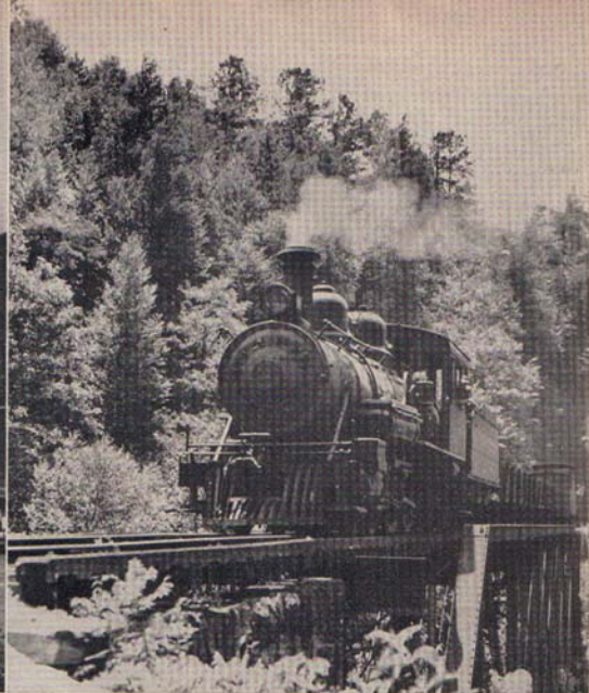
The Ten-Wheeler has just emerged from a tunnel, and the fireman and head brakeman are inspecting the train on the brief stretch of open track across this inverted truss bridge. The tunnel was approached at both ends by bridges; construction of the line through Doe River Gorge was not easy.
